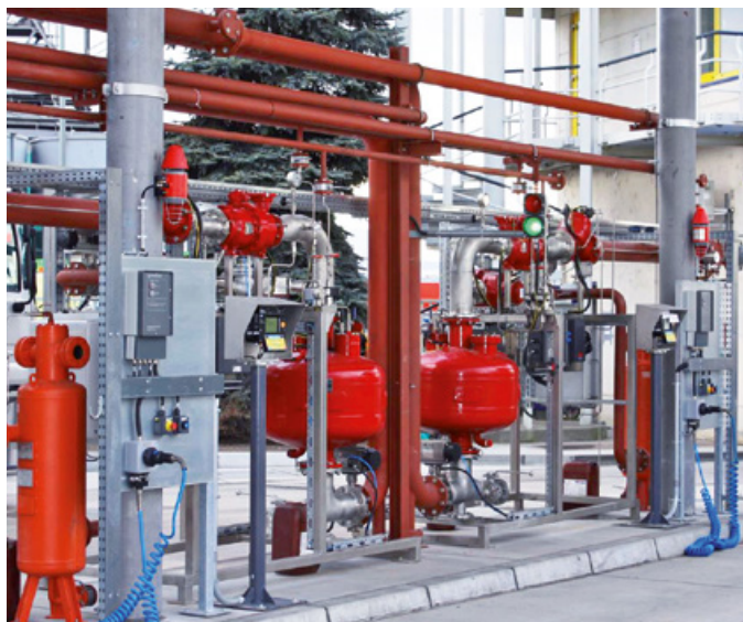
↑ CMS: Compact Metering Skid
